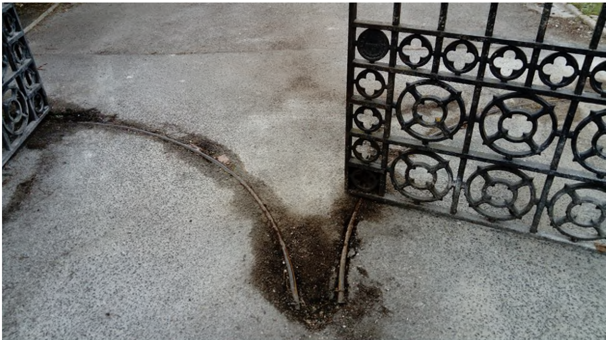
Figure 2 - Gates and wheel tracks
