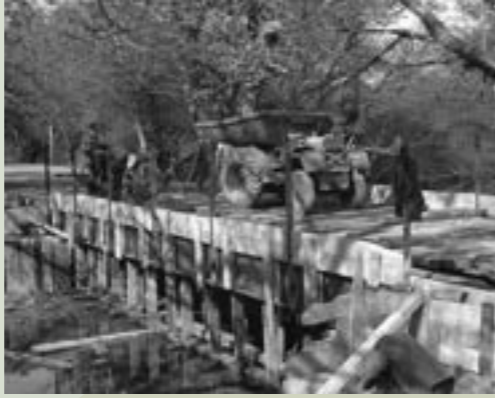
Working on widening and strengthening Mill Road bridge Brockenhurst during build up to D Day ©IWM
